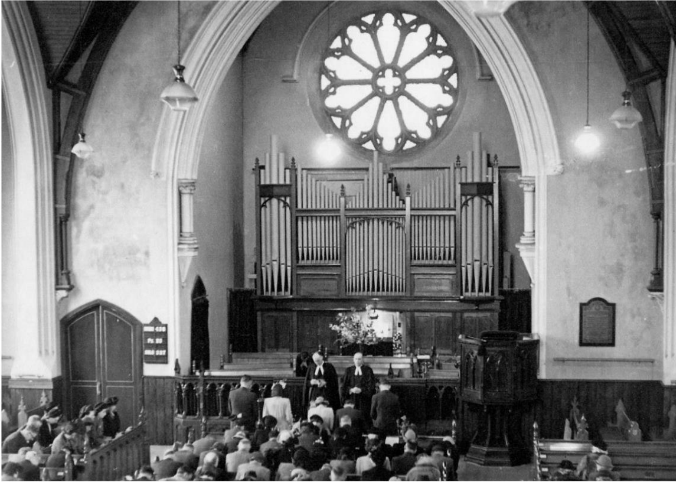
Church interior, April 1948.
